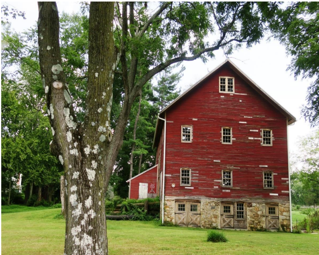
Restored Old Barn
