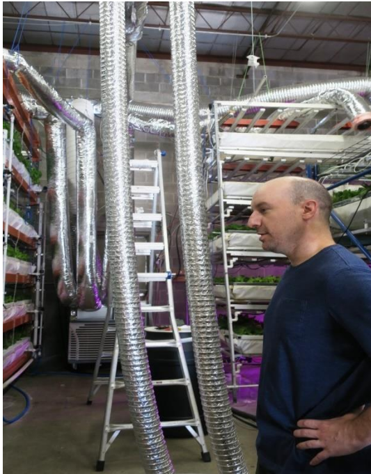
Dominic Shows Us His Ducts
